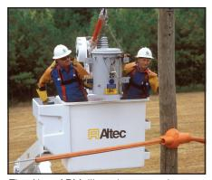
The Altec ARM Jib makes removing and installing transformers Safer and Smarter<sub>®</sub>.
